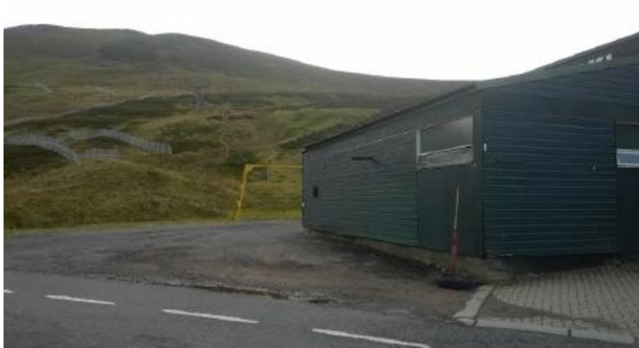
Figure 3 (a) Photograph of existing drive-station and chairlift
