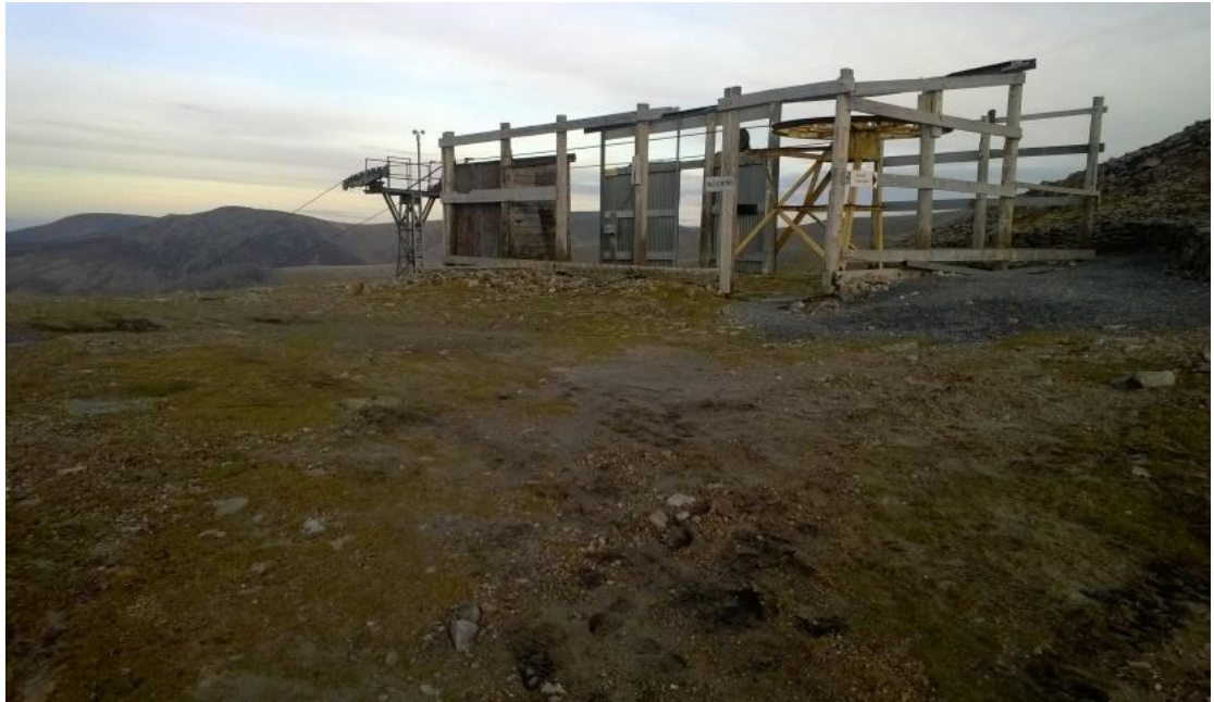
Figure 4 (a) Photograph of existing drive-station
